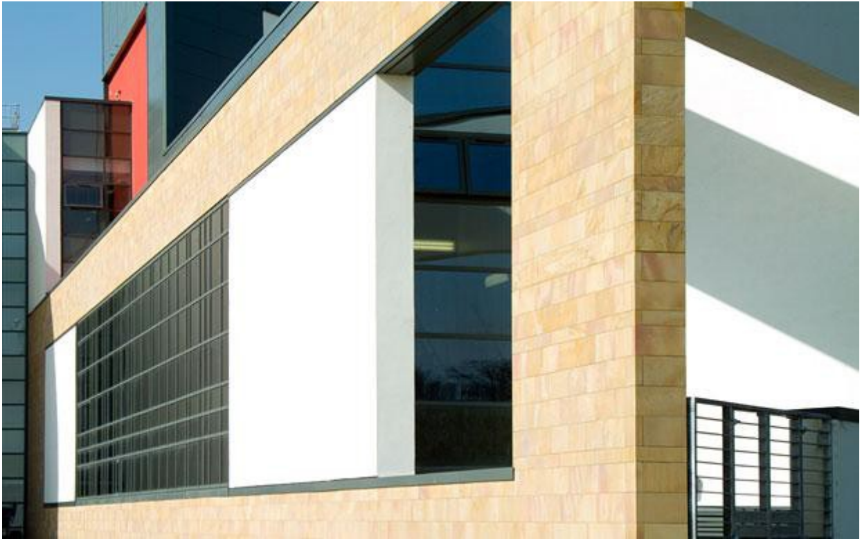
Forth Valley Royal Hospital Exterior
